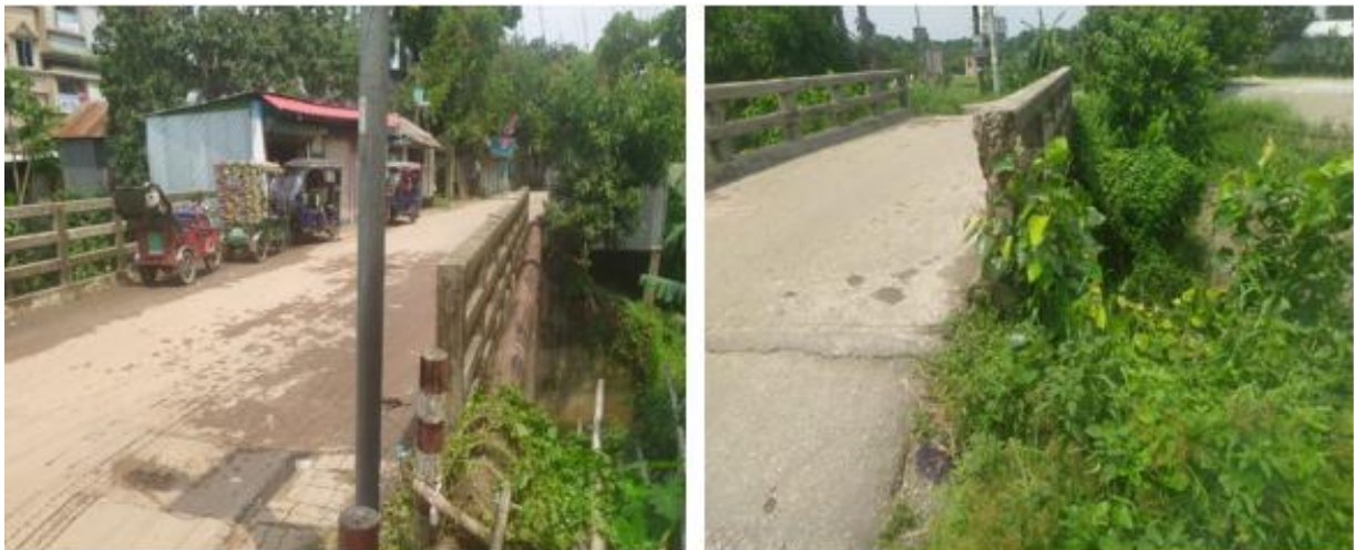
Photographs 2.2.2: Current Situation of the Outfall at Subproject Site
