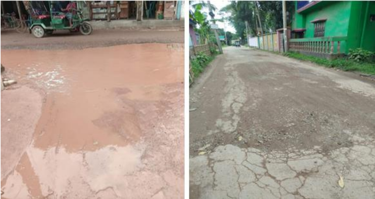
Photographs 2.2.1: Existing Road Condition of the Subproject Site
