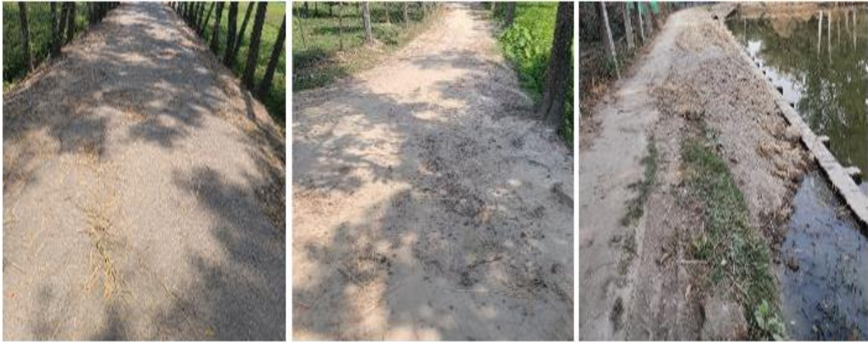
Photographs 2.2.1: Existing Road Condition of the Subproject Site
