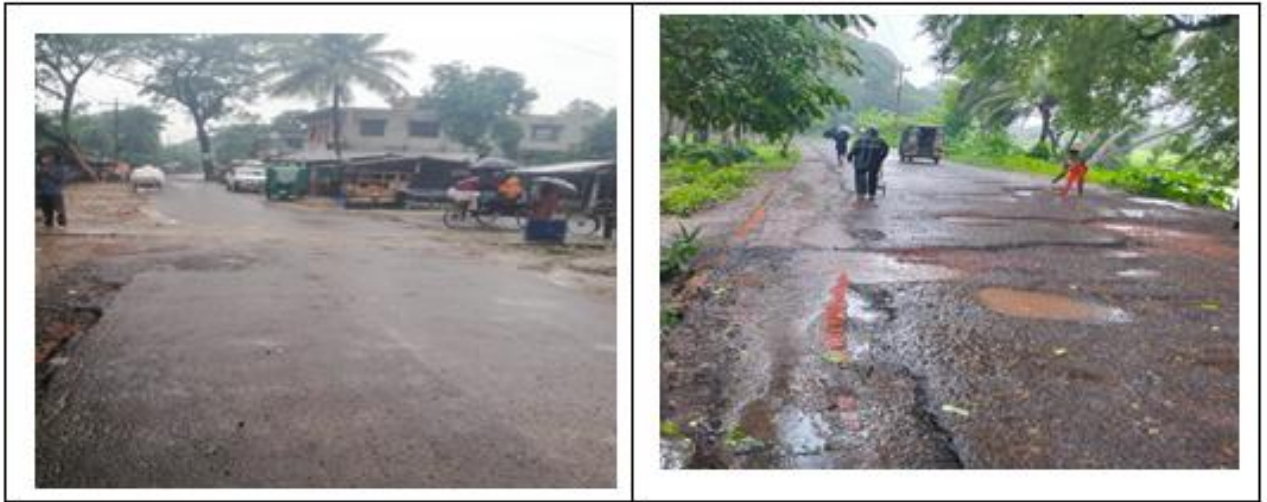
Photograph 2.2.1: Existing Road Condition of the Subproject Site
