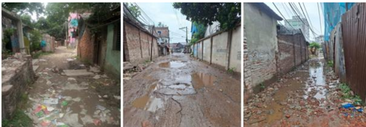
Photographs 2.2.1: Existing Road Condition of the Subproject Site
