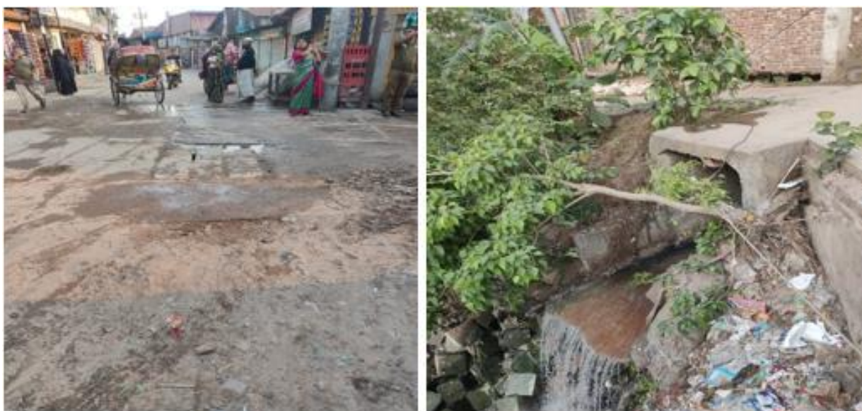
Photographs 2.2.2: Current Situation of the Outfall at Subproject Site
