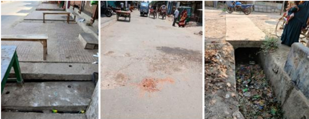
Photographs 2.2.1: Existing Road with Drain Condition of the Subproject Site
