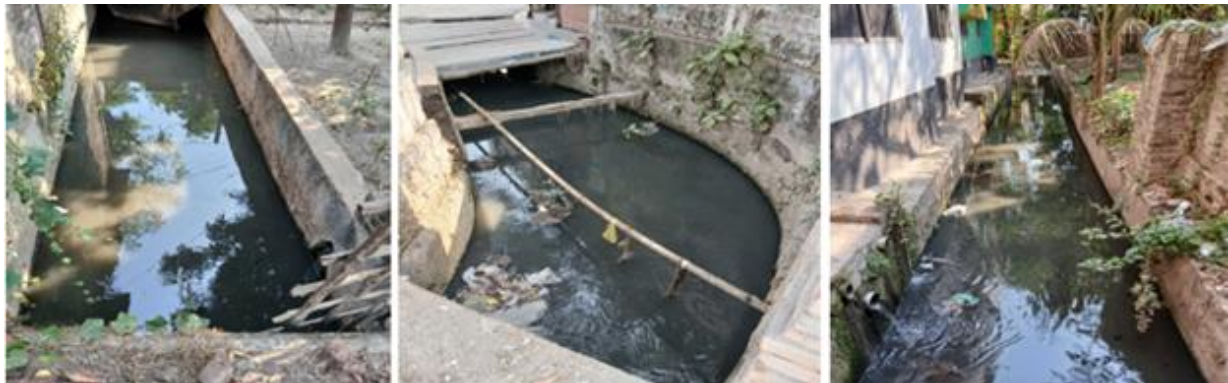
Photographs 2.2.2: Current Situation of the Outfalls at Subproject Site
