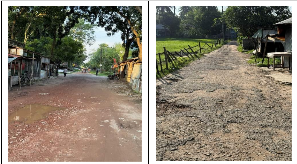
Photograph 2.2.1: Existing Road Condition of the Subproject Site
