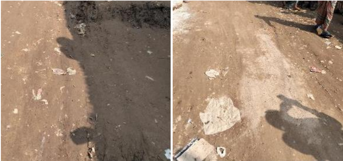
Photographs 2.2.1: Existing Road Condition at the Subproject Site
