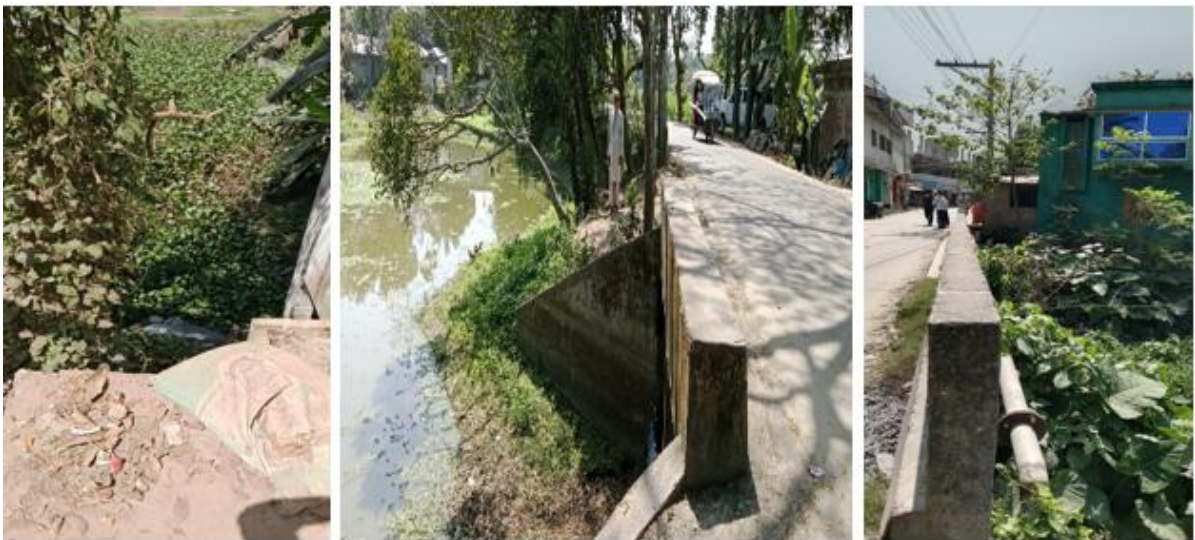
Photographs 2.2.2: Current Situation of the Outfalls at Subproject Site
