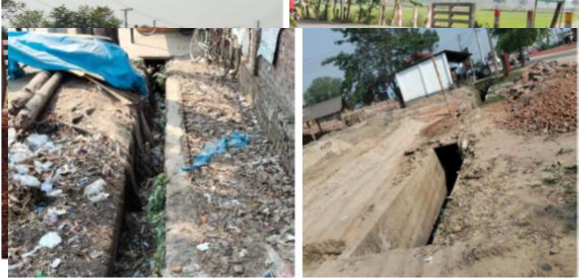
Photographs 2.2.1: Existing Road Condition of the Subproject Site
