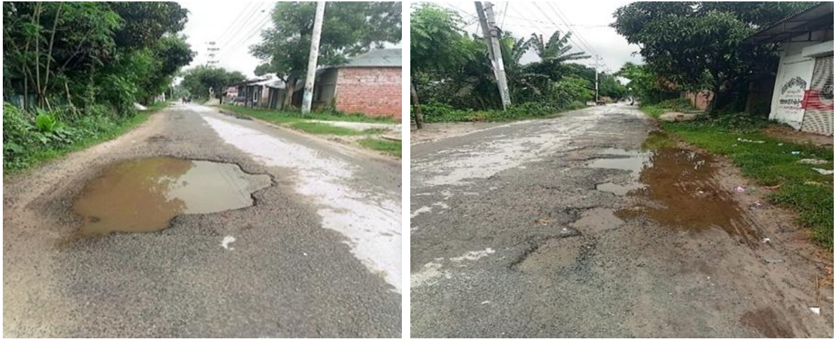
Photograph 2.2.1: Existing Road Condition of the Subproject Site
