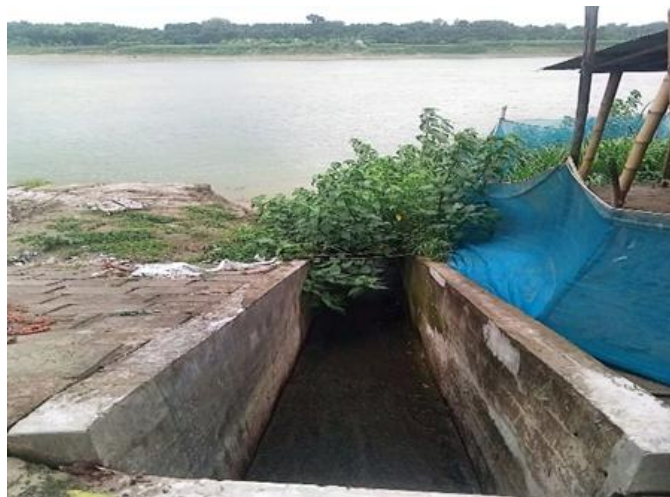
Photograph 2.2.3: Current Situation of the Outfalls at Subproject Site
