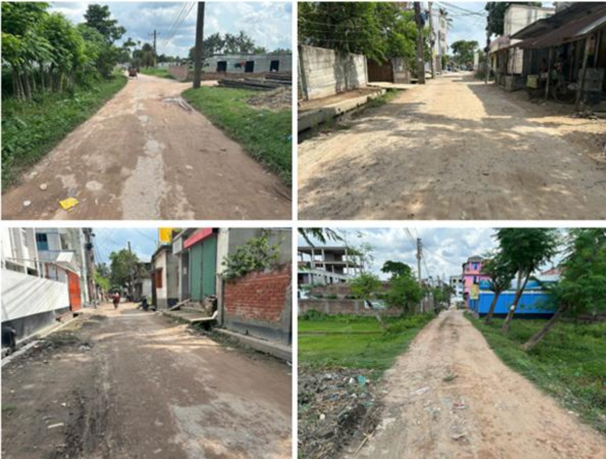
Photographs 2.2.1: Existing Road Condition of the Subproject Site
