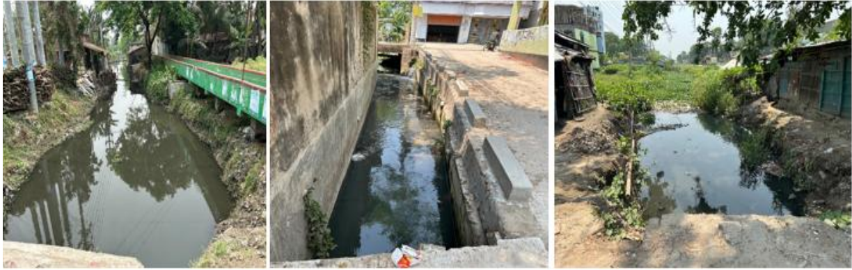
Photographs 2.2.3: Current Situation of the Outfall at Subproject Site
