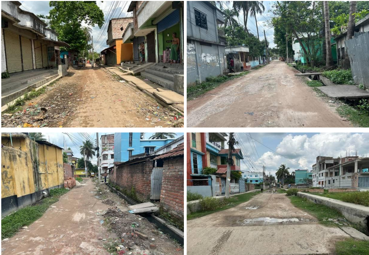
Photographs 2.2.2: Existing Road with Drain Condition of the Subproject Site
