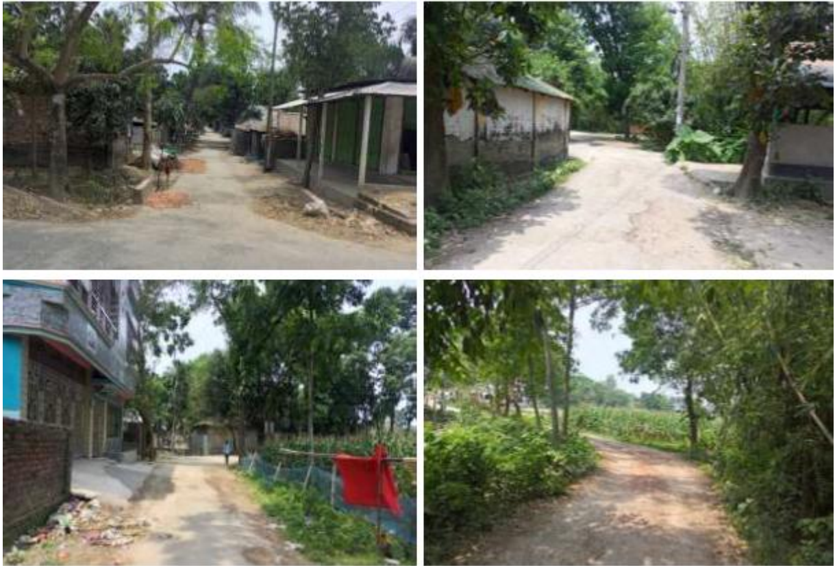
Photographs 2.2.1: Existing Road Condition of the Subproject Site
