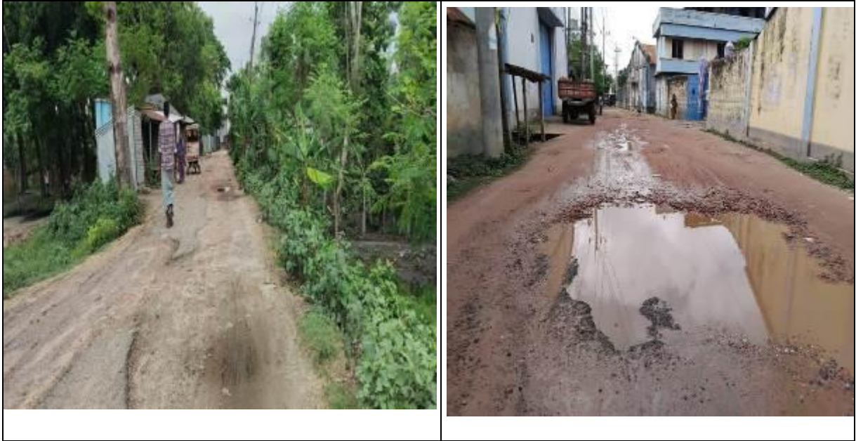
Photograph 2.2.1: Existing Road Condition of the Subproject Site
