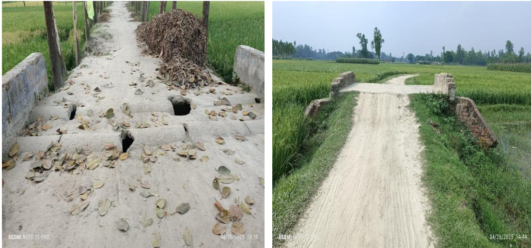
Photographs 2.2.2: Current Situation of the Existing Culverts at Subproject Site
