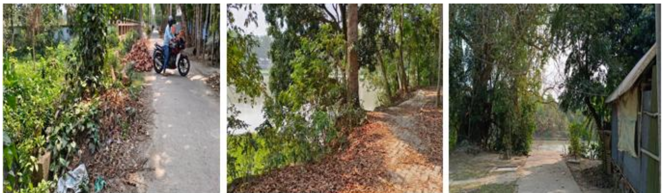
Photographs 2.2.3: Current Situation of the Outfalls at Subproject Site
