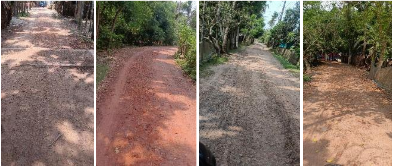
Photographs 2.2.1: Existing Road Condition of the Subproject Site
