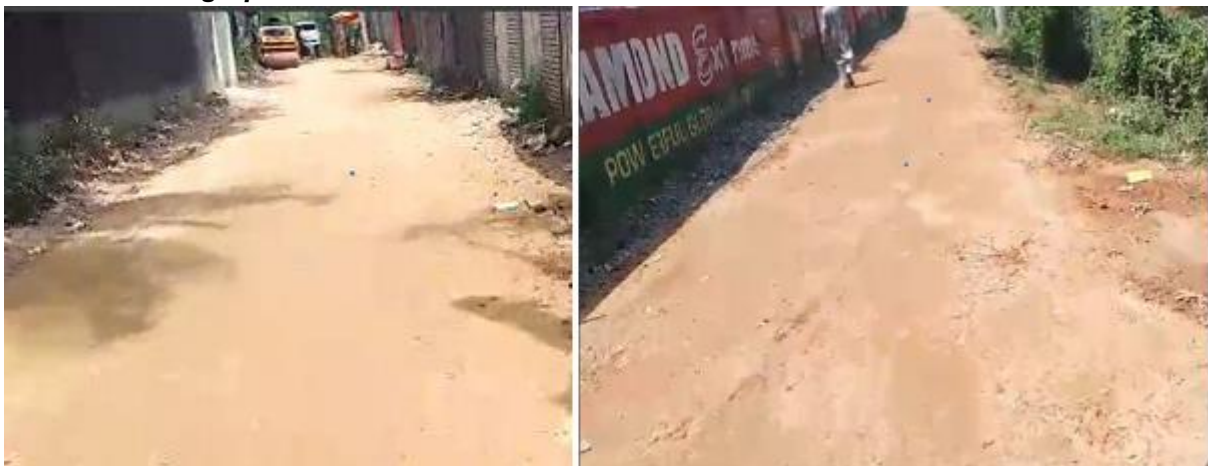
Photographs 2.2.1(a): Existing Road Condition of the Subproject Site
