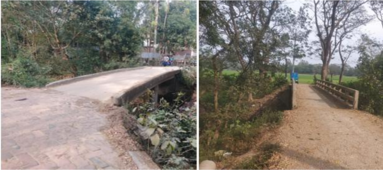
Photographs 2.2.1(b): Existing Road Condition with Culverts of the Subproject Site
