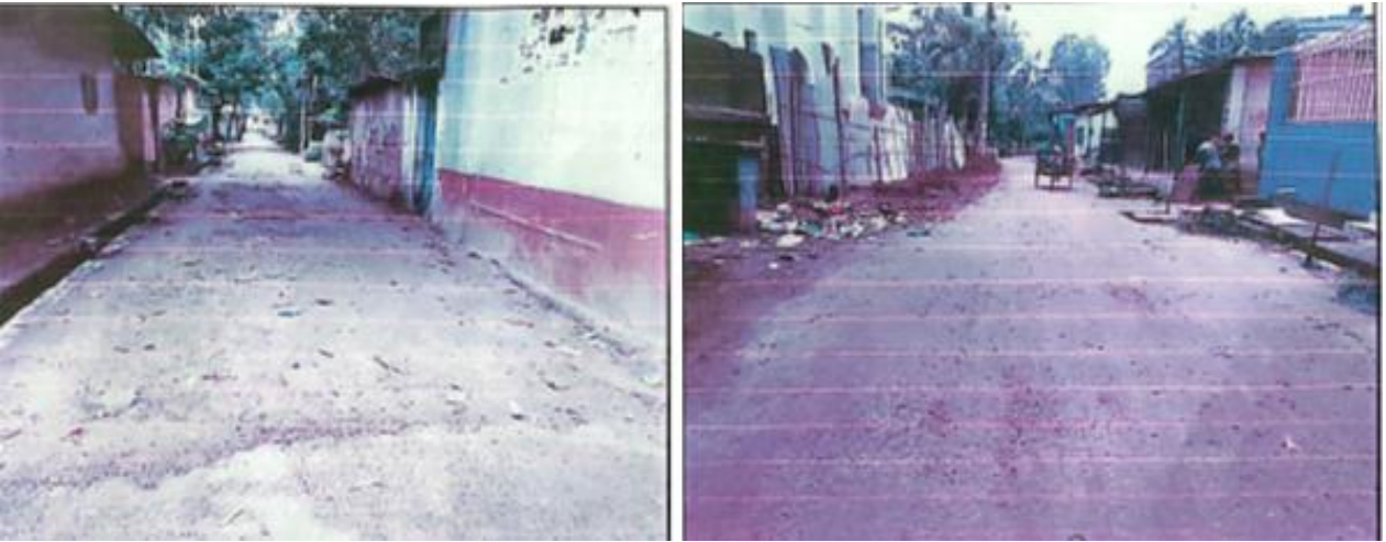
Photographs 2.2.2: Existing Road with Drain Condition of the Subproject Site
