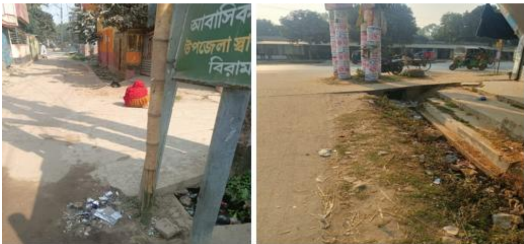
Photographs 2.2.3: Current Situation of the Outfall (Existing Drain) at Subproject Site
