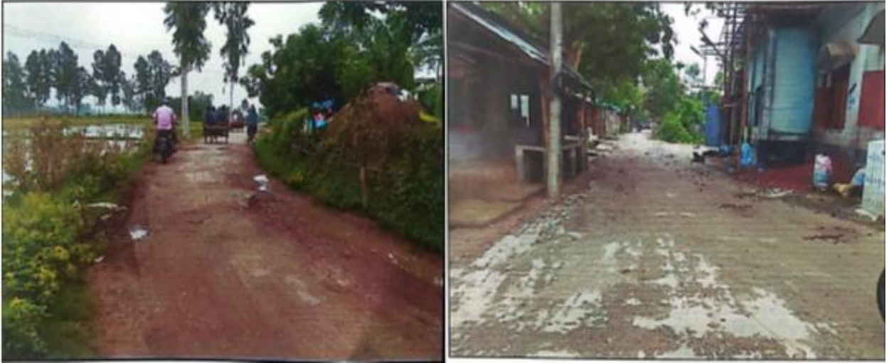
Photographs 2.2.1: Existing Road Condition of the Subproject Site
