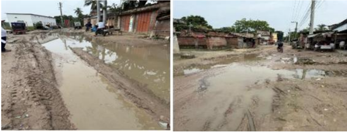
Photograph 2.2.1: Existing Road and drain Condition of the Subproject Site
