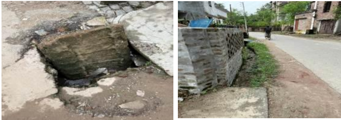
Photograph 2.2.2: Existing Road and drain Condition of the Subproject Site
