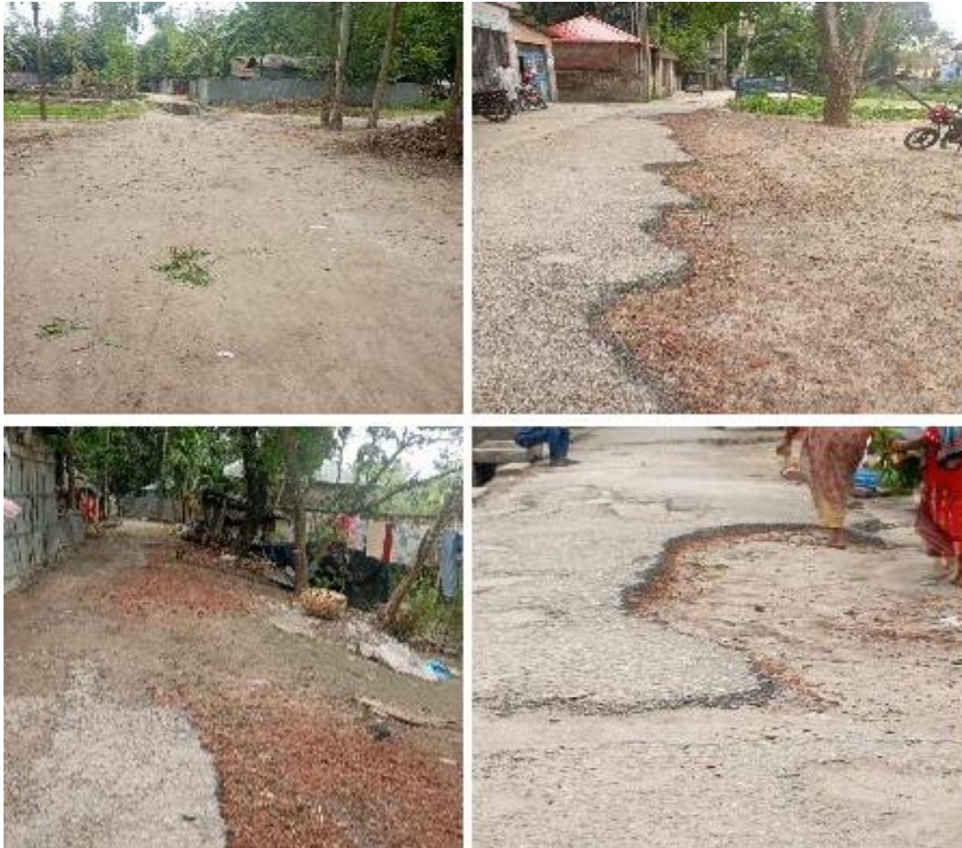
Photographs 2.2.1: Existing Road Condition of the Subproject Site
