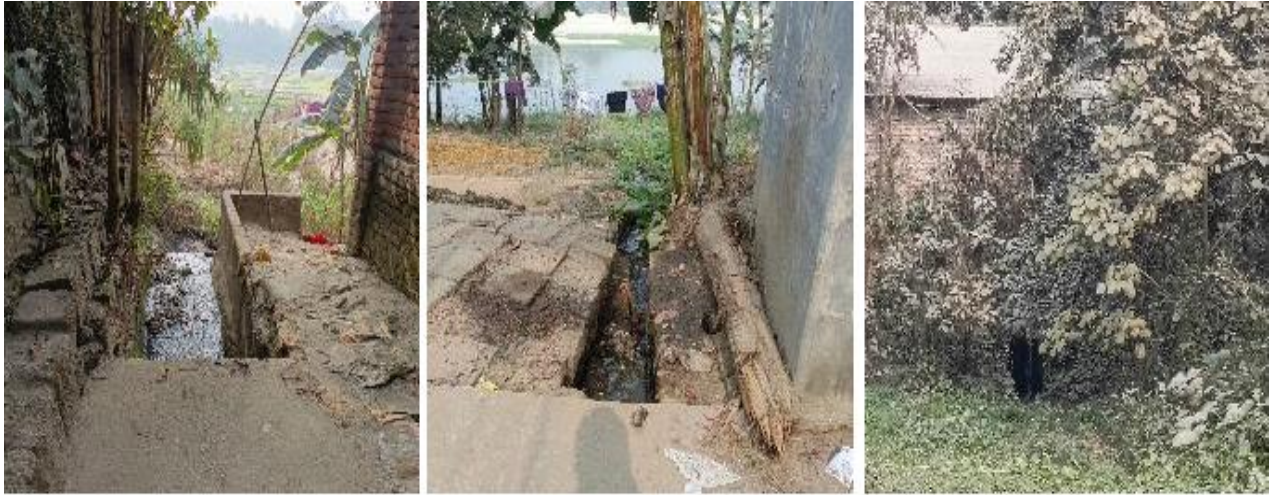
Photographs 2.2.3: Current Situation of the Outfall at Subproject Site
