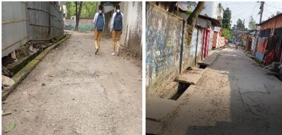
Photographs 2.2.2: Existing Drain Condition of the Subproject Site
