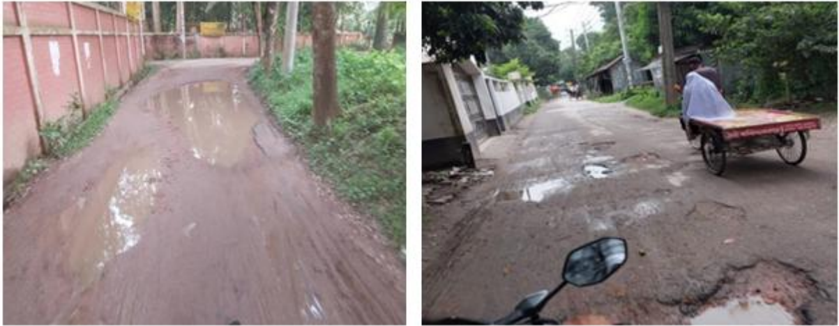
Photograph 2.2.1: Existing Road Condition of the Subproject Site
