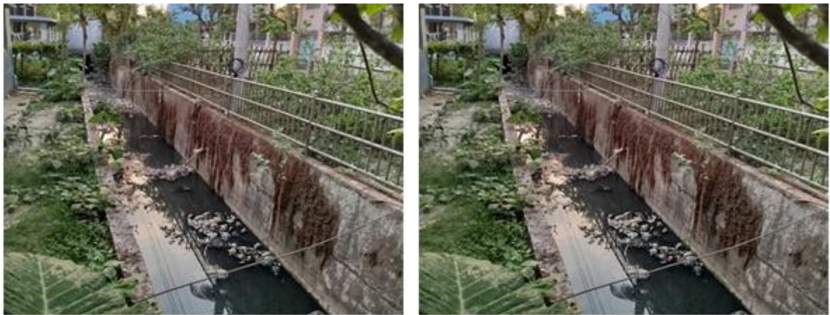
Photograph 2.2.2: Existing Drain Condition of the Subproject Site
