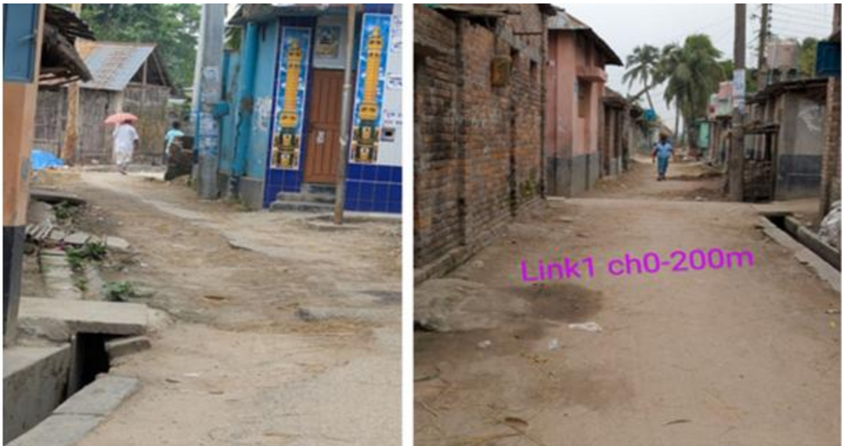
Photographs 2.2.2: Existing Drain Condition of the Subproject Site
