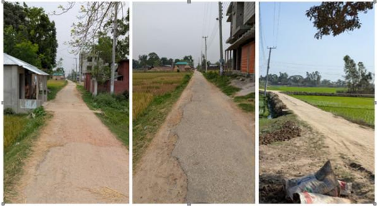
Photographs 2.2.1: Existing Road Condition of the Subproject Site
