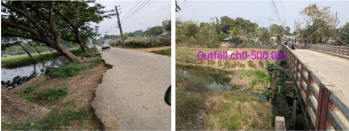
Photographs 2.2.3: Current Situation of the Outfall at Subproject Site
