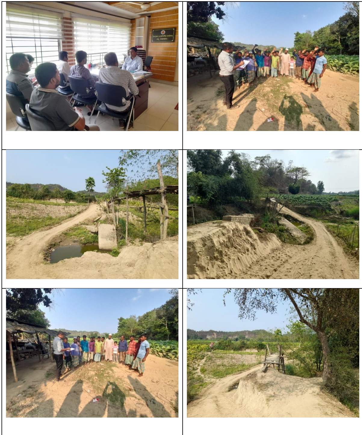
Figure: Present condition of the proposed location for 40m RCC Arch Bridge at ch 600 on Zarulia Chari on Moiskum Bridge - Mokters Bari Road ID: 4226640229 (Package no: HELP-COX/BR-1) (Ramu Upazila)
