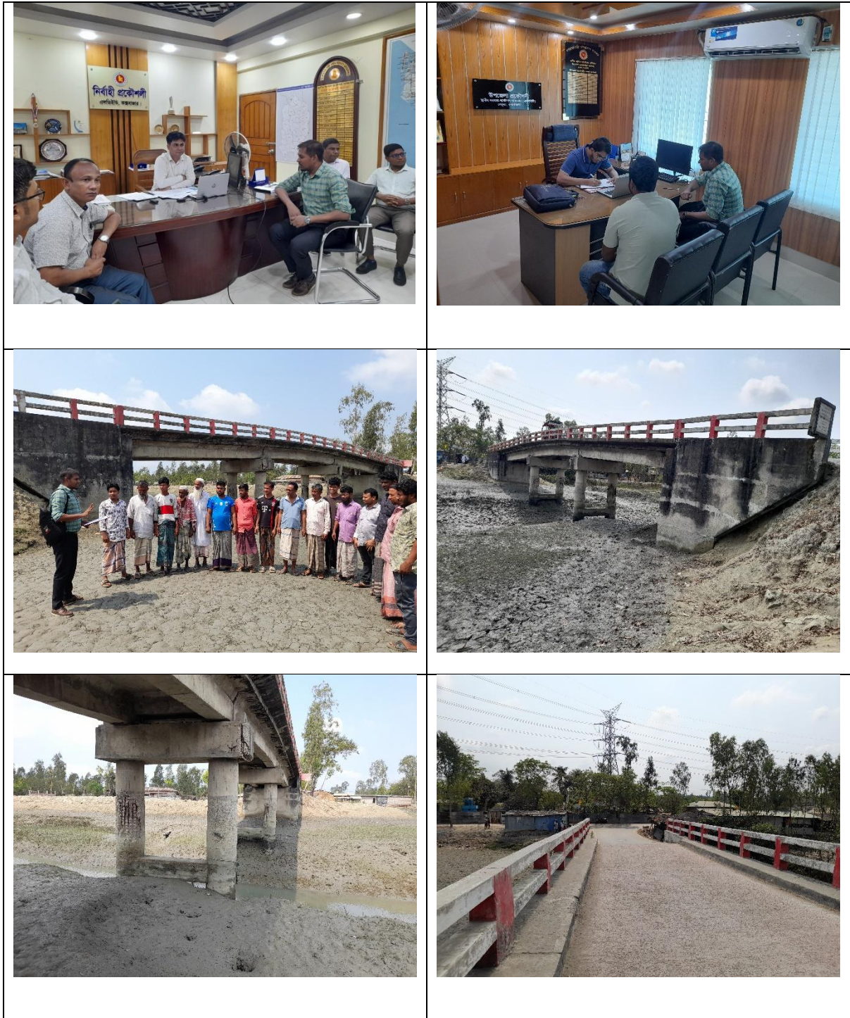
Figure: Present condition of the proposed location for 65m Long RCC Bridge at ch 1520 on Rekuia to Arabshah Bazar via Rajakhali Sabuj Bazar road ID: 422952002 (Package no: HELP-COX/BR-1) (Pekua Upazila)
